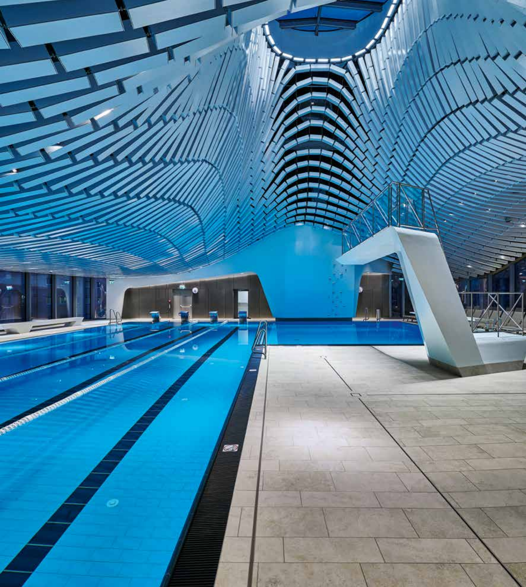
Paracelsus Bad & Kurhaus, Salzburg, Austria / Architect: Berger + Parkkinen / Series: Pool edge systems Wiesbaden, Savona / Photo: Christian Richters
